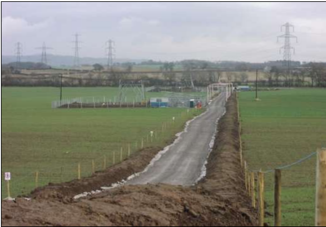
Figure 5.5 Temporary Stone Access Track with Pylon Construction Area
