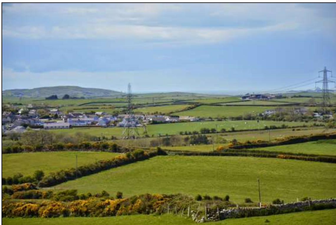
Figure 8.2 Looking West Towards Tregale with Existing Overhead Line in the Foreground
