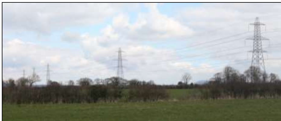
Existing L6 Tower
