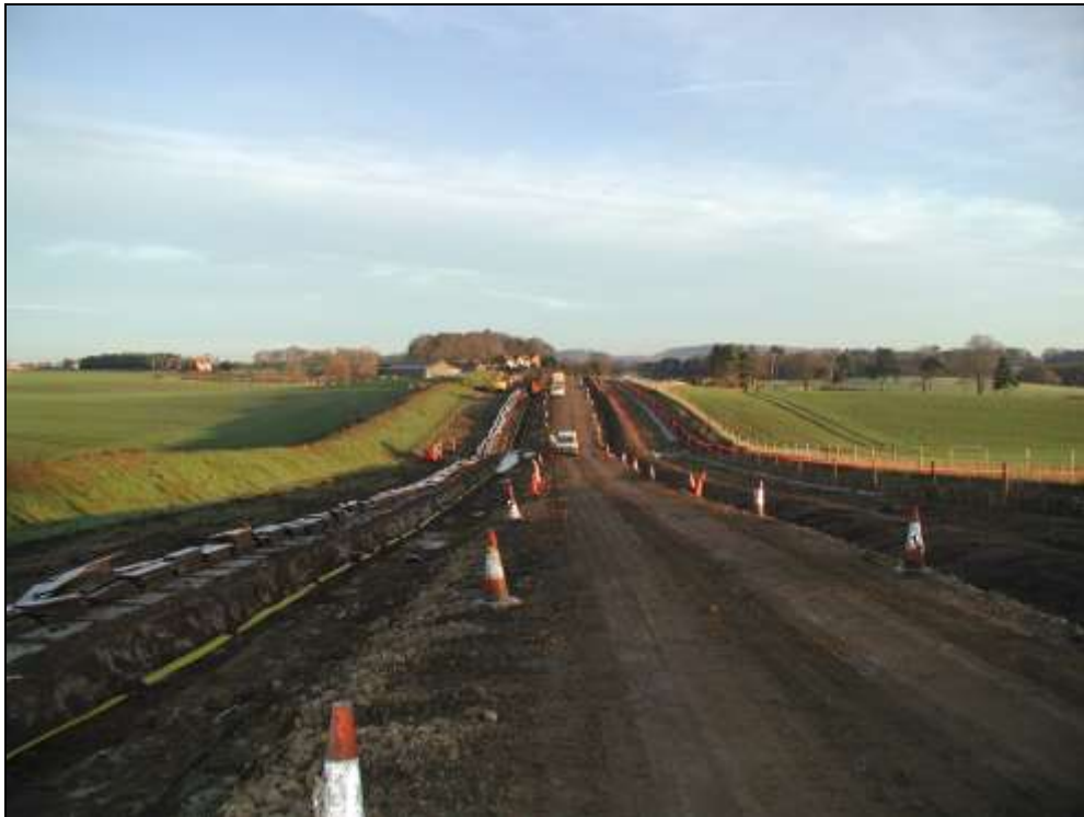
Figure 5.9 Construction Working Area during Underground Cable Laying
