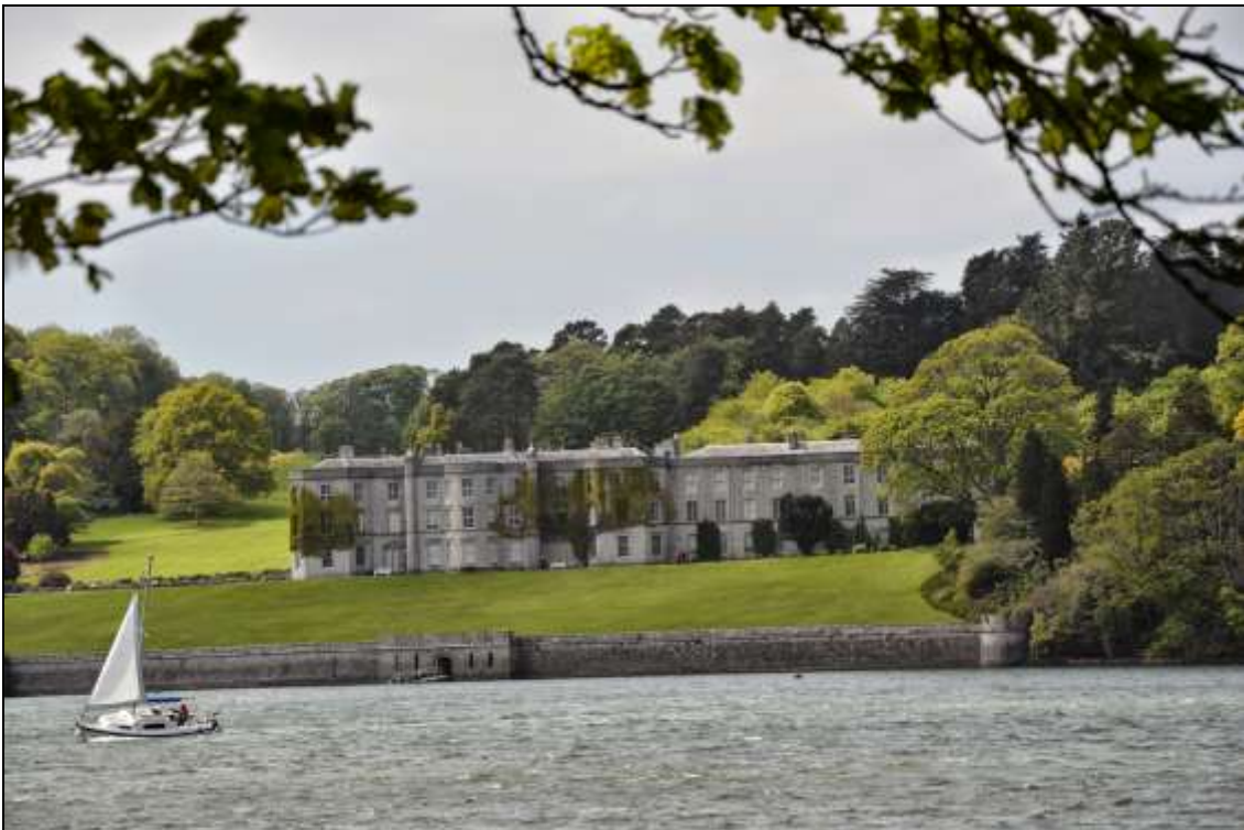
Figure 9.9 Plas Newydd Grade I Listed House and Registered Park and Garden
