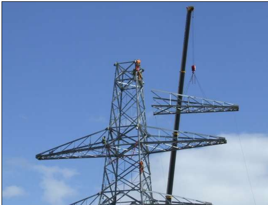
Figure 5.6 Crane Assembling a Tower
